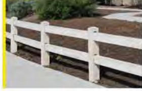
TWO RAIL CONCRETE FENCE (3')
