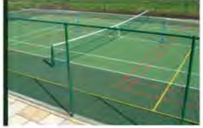
TENNIS COURT/PICKLEBALL VINYL COATED CHAIN LINK FENCE (10')
