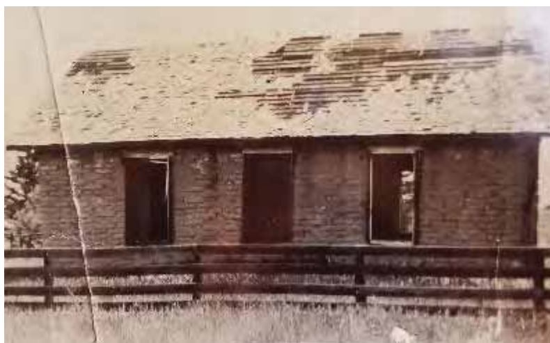
Figure 7. Estrella Adobe Church, prior to restoration (Paso Robles Historical Society)
