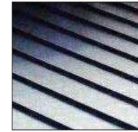
STANDING BATTAN METAL ROOF
