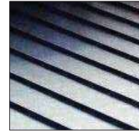
STANDING BATTAN METAL ROOF
