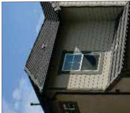
Siding terminating at outside corner where miter boards are used
