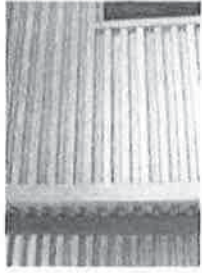
SIDING: 1 1/2" DEEP ALUMINUM WALL PANEL (MATRIX MX1.0 24 GA.) MFR: MORIN, COLOR: GALVALUME TO MATCH EXISTING
