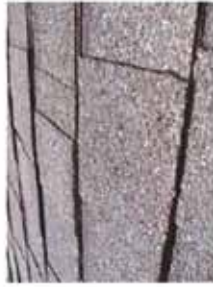
ASPHALT SHINGLE ROOFING
