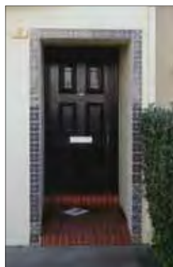
Recessed door with tile
