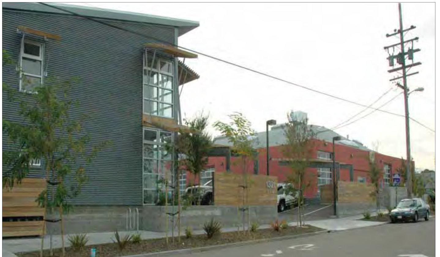
Continuous low concrete wall with taller wooden screens define the property edge. A break is made for bicycle storage and access to the parking lot.
