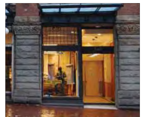
The wall below the base cornice changes from brick and is anchored with heavy masonry columns
