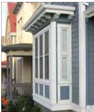
New construction: one story square bay with brackets
