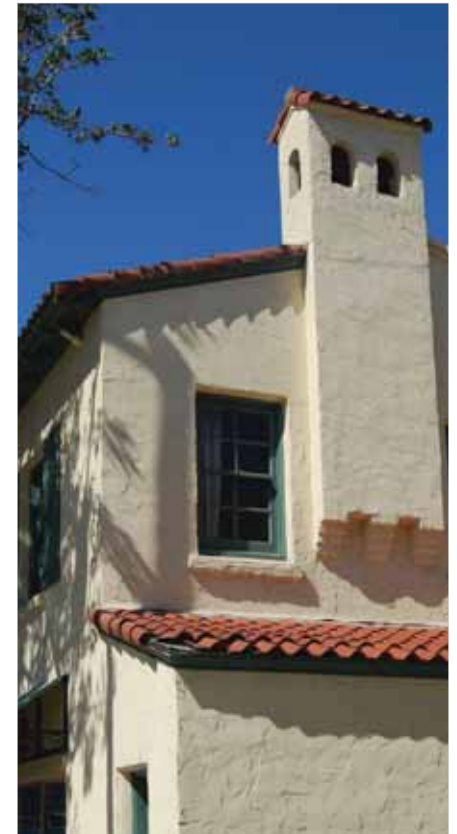
Chimney with corbelled base engaged in the side gable
