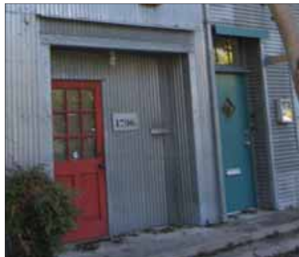
Swing doors with windows
