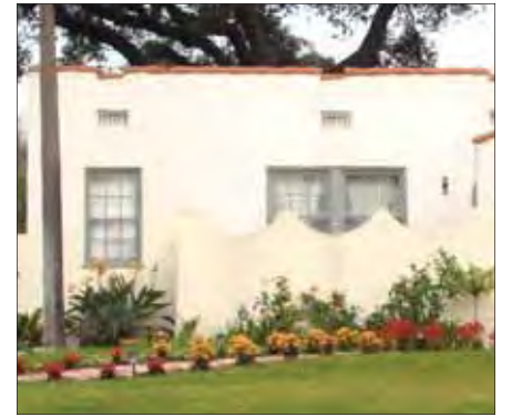
Parapet with flat roof
