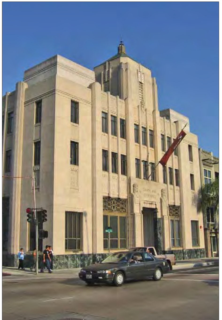
Rectangular massing with central and corner tower elements. Pilasters run from base of the building to the top.
