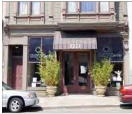
Storefront with awning; entry to second story at left
