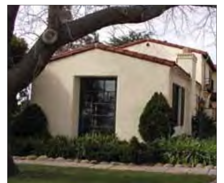
Stucco walls with windows recessed in punched openings. Walls have no base.
