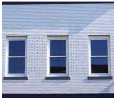
Double hung windows set in simple brick frame
