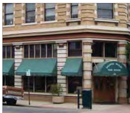
The wall below the base cornice is composed of a combination of materials, different from the primary wall above
