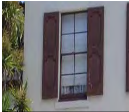
Fixed window with operable shutters and stucco sill
