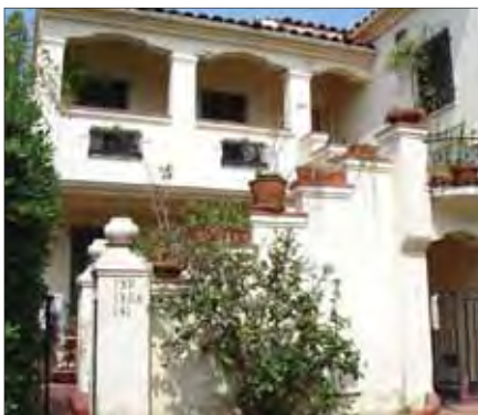
Exterior stair from courtyard
