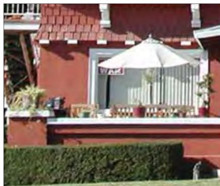
Concrete base finished with stucco
