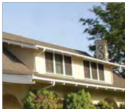
Shed dormer with asphalt shingles and deep overhang
