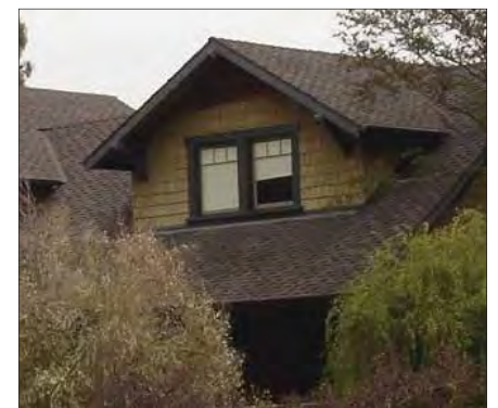
Cross gable dormer with wood shingles and deep overhang supported by brackets
