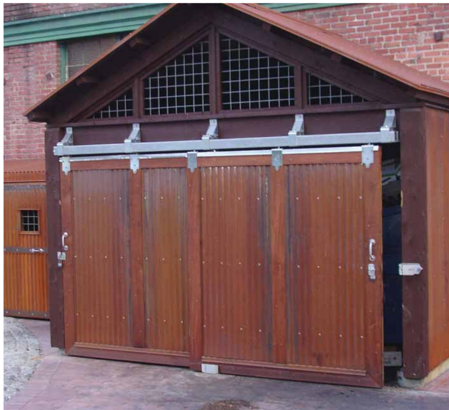
Single slider garage door with external track
