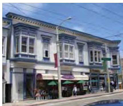
Large massing with elaborate cornice and bay windows; transoms at the corner
