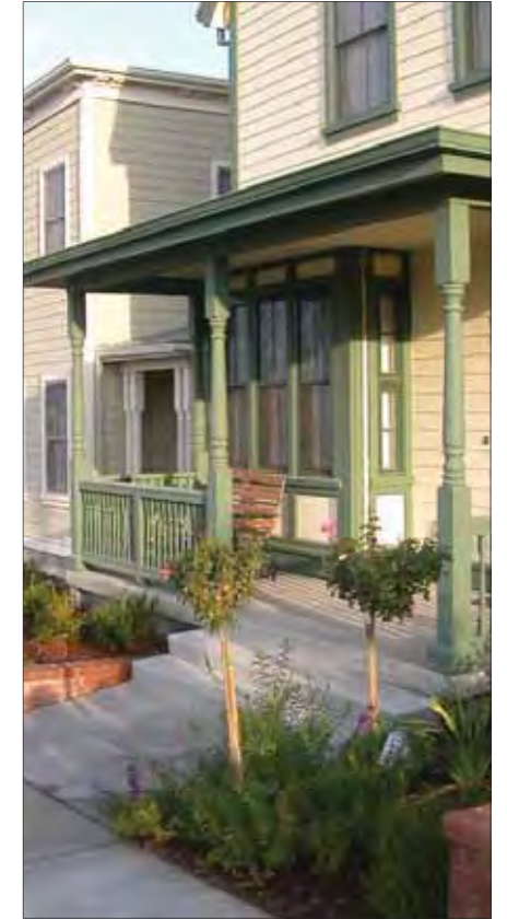
Porch enclosing a square bay window
