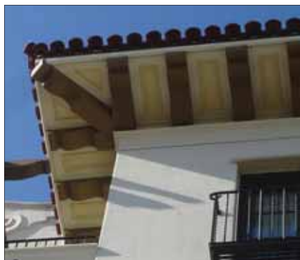
Open eave with exposed rafter tails and simple coffering in soffit
