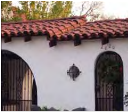
Sloped tile roof
