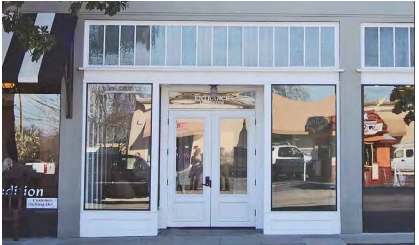
Recessed entry with a transom window across entire storefront. Wood paneling at base of storefront
