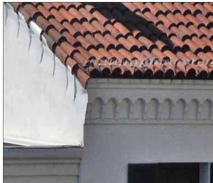
Closed eave with stucco detailing
