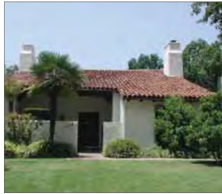
Sloped tile roof
