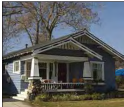
Gable end with gable end porch
