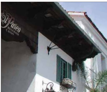
Expressed rafters, broad eave
