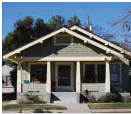
Roofs parallel to street
