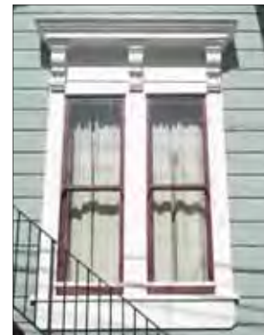
Ganged, double-hung window with decorative brackets
