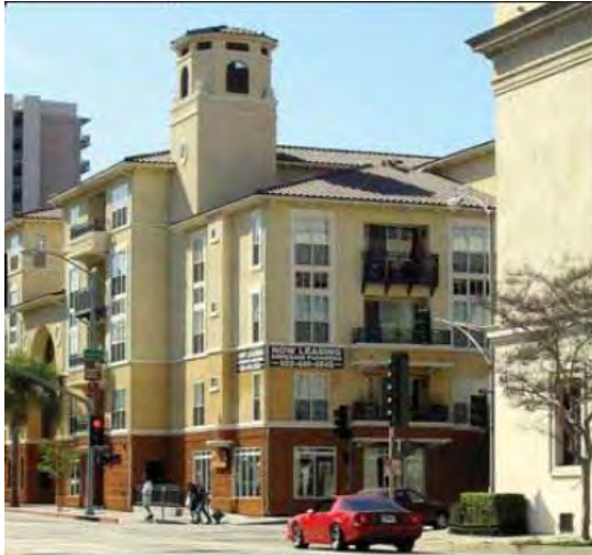
Illustrative Photo: Stacked dwelling with on-street access
