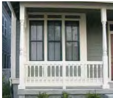
Turned posts and railing
