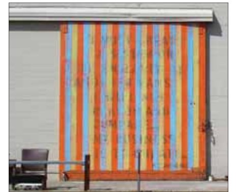
Single slider garage door with external track
