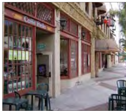
Recessed storefront doors with transom windows flush with storefront windows.
