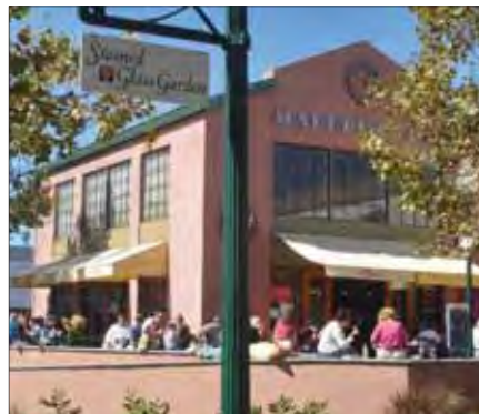
Gable end warehouse with shopfront
