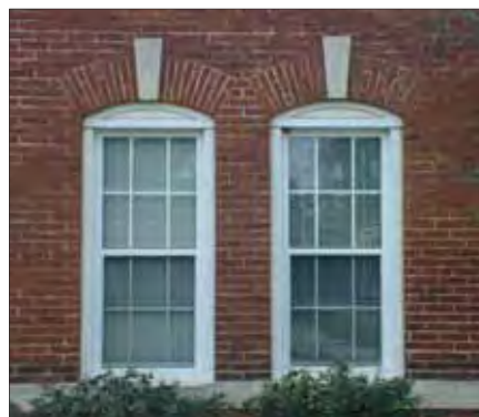
Double hung windows set in an arched-brick frame and keystone
