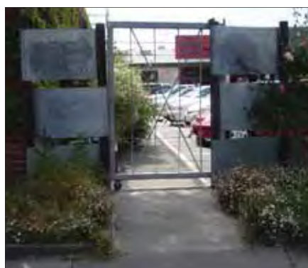
Gate and fence screen parking lot
