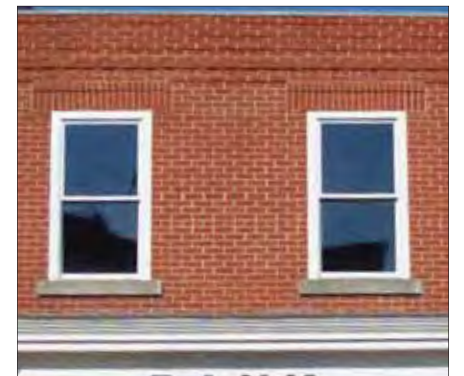
Double hung windows set in simple brick frame
