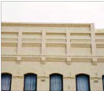
Corbelled, painted brick parapet
