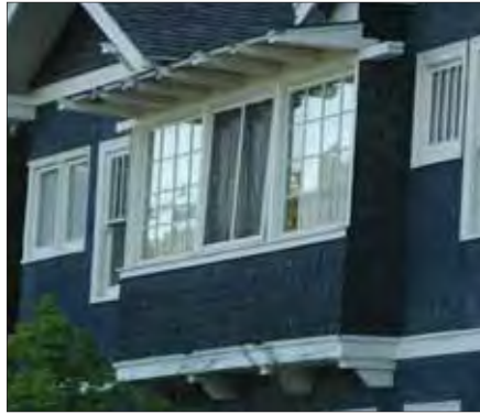
Square side bay supported by heavy brackets
