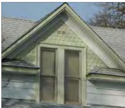
Vertically proportioned windows tucked into a gabled dormer
