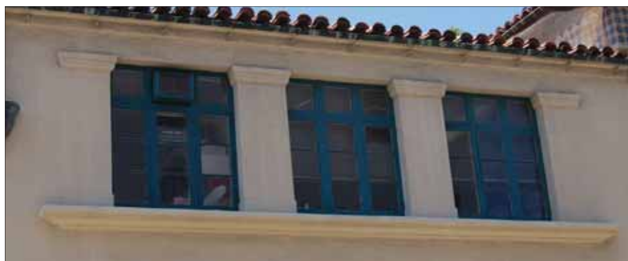
Three part bay of windows divided by stucco pilasters, also with three part divisions within each window bay
