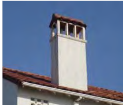
Chimney with openings and tile roof
