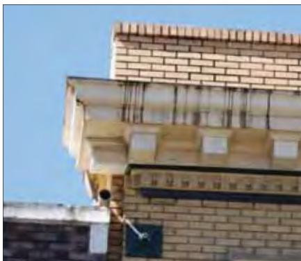
Attached formal cornice
