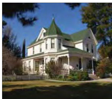
Example of a high-style victorian with an octagonal corner turret which the porch engages
