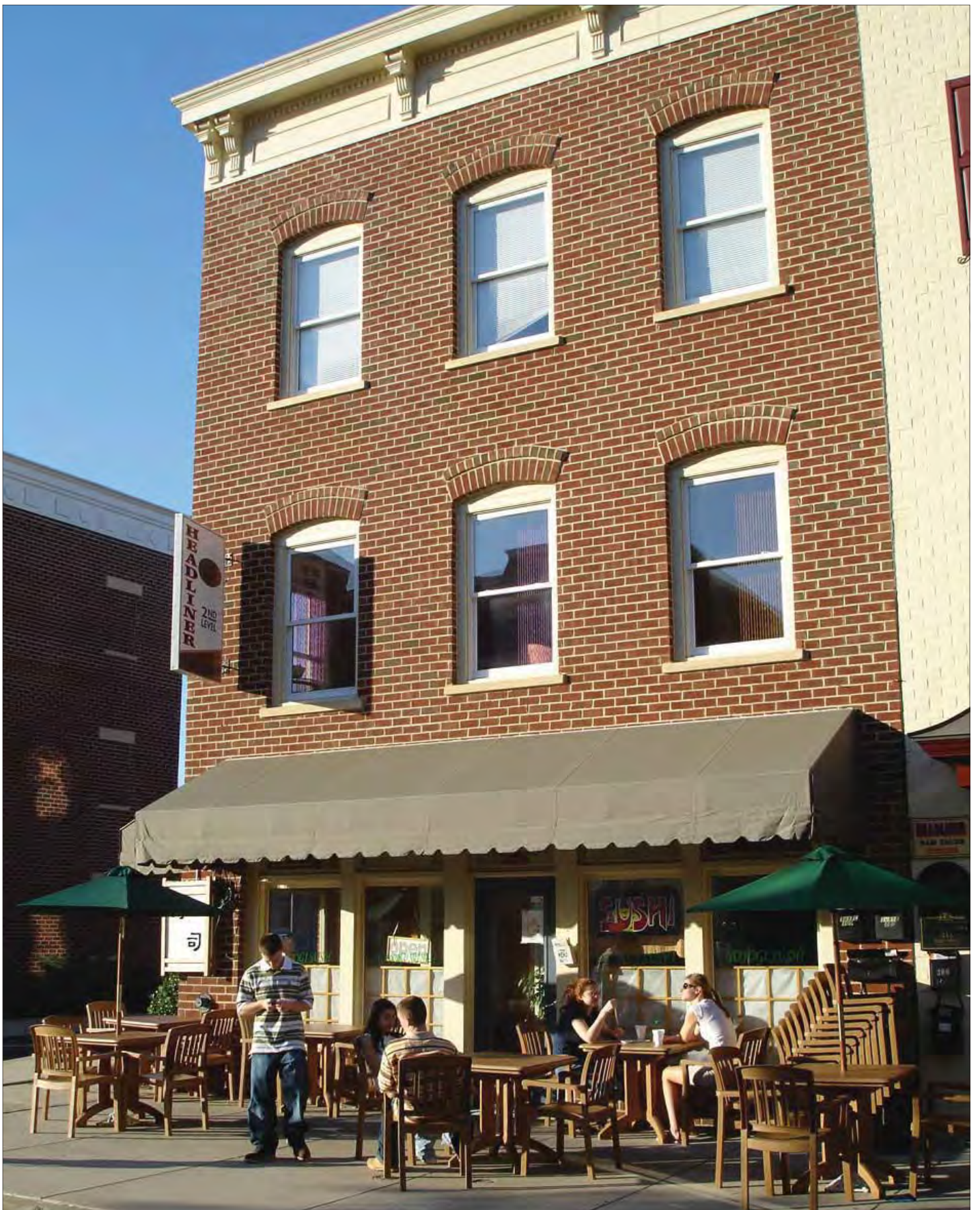
New construction of a well-proportioned and detailed Main Street building. The building is designed as a simple wall plane with appropriate proportion of wall to window opening, depth in the windows, and cornice scale and detail.
