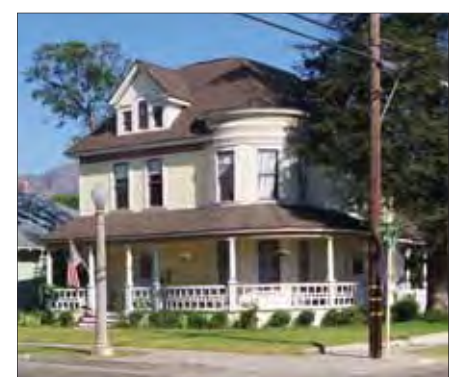
Example of a high-style victorian with a round corner turret which the porch engages
