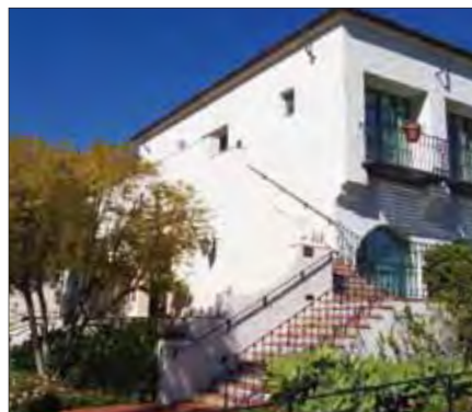
Exterior stair from plaza
