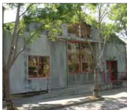
Gable end warehouse with loading dock frontage
