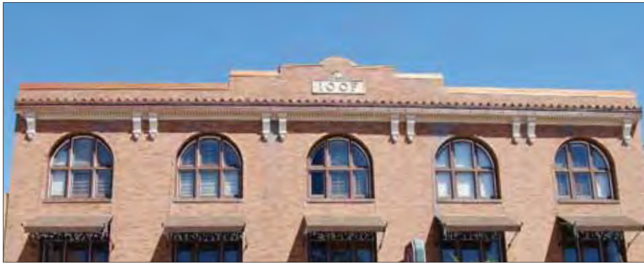
Continuous parapet with central detail and attached cornice
