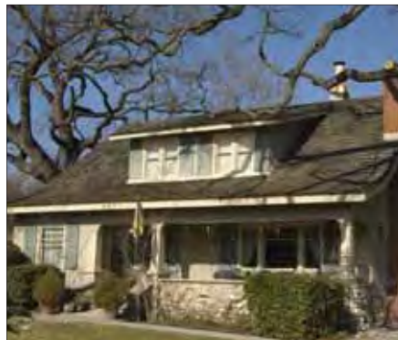
Side gable with shed dormer
