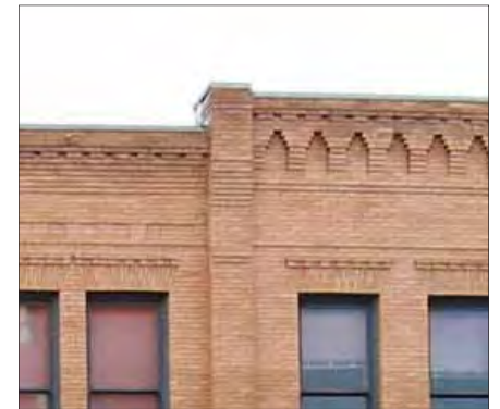
Corbelled brick parapet steps up for hierarchy
