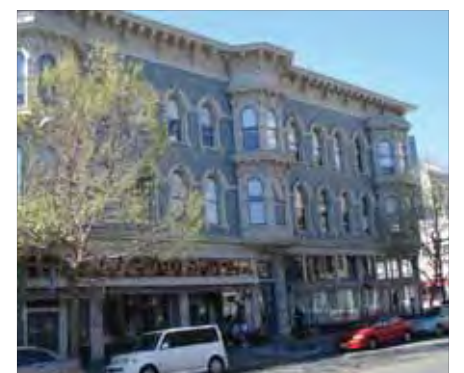
Large massing with elaborate cornice, two-story bay windows and detailed storefronts
