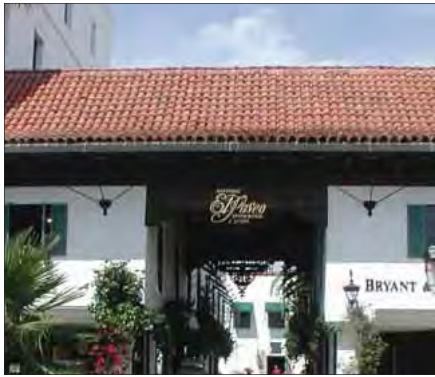
Sloped tile roof
