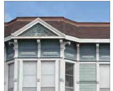
Tall cornice with small gable
