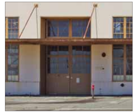
Single slider garage door with external track
