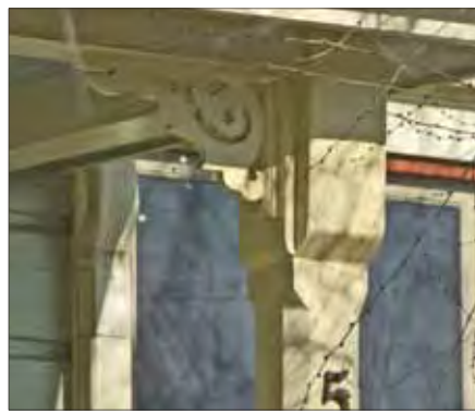
Chamfered square posts with decorative bracket
