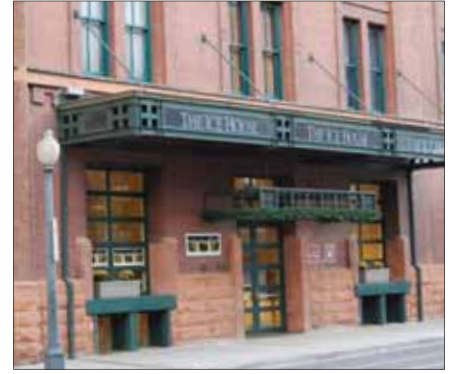
Canopy at commercial frontage
