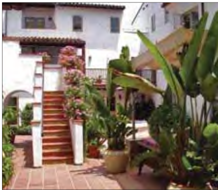
Exterior stair off of a courtyard
