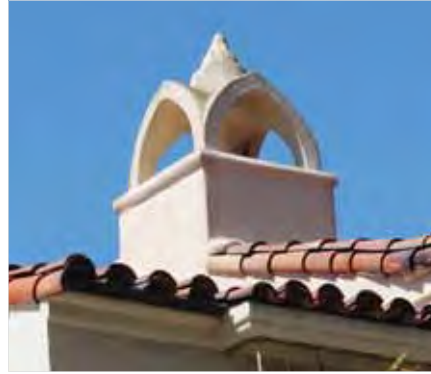
Chimney with ornamental top
