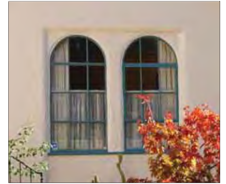
Double arch windows
