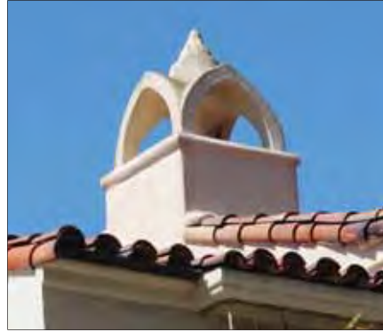
Chimney with ornamental top
