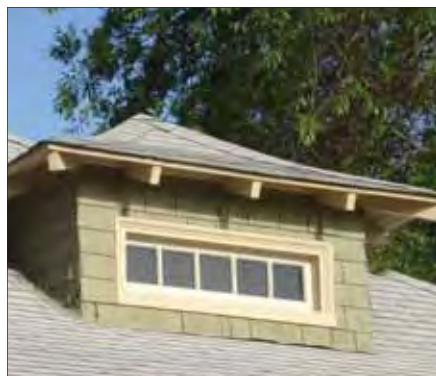
Hipped dormer with asphalt shingles and deep overhang
