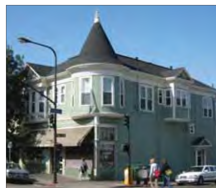
Round turret at building corner over a commercial storefront
