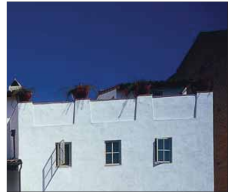
Parapet as extension of exterior wall
