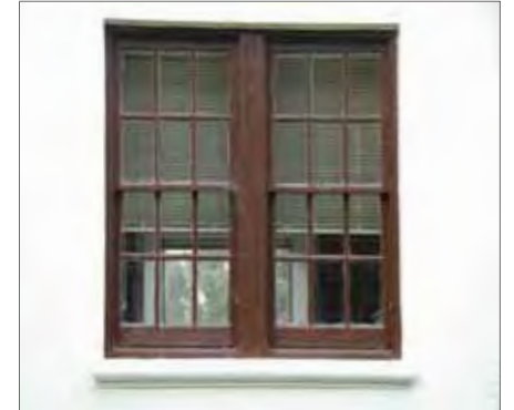
Wood casement window with vertically proportioned panes and a stucco sill
