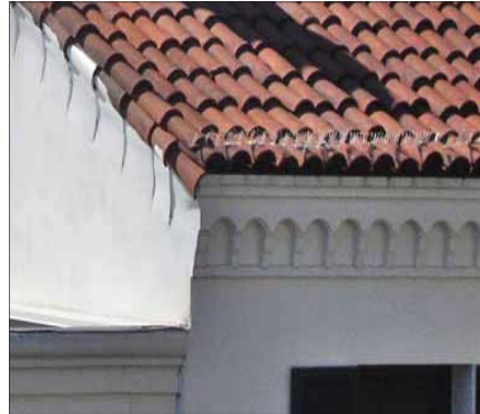
Closed eave with stucco detailing
