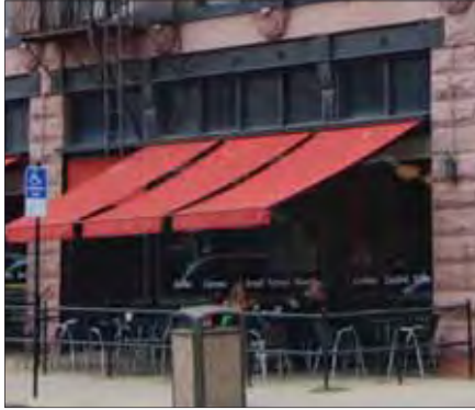
Awning that is part of storefront and hinges below the transom windows
