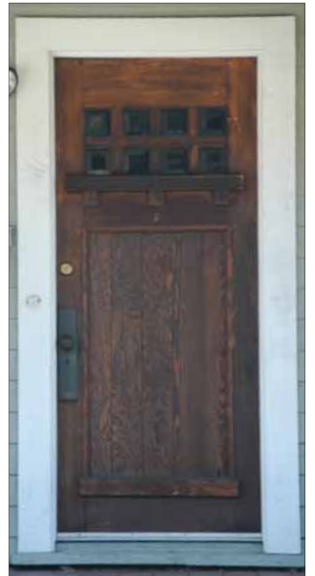
Simple, paneled door with upper-door windows and a shelf below the window
