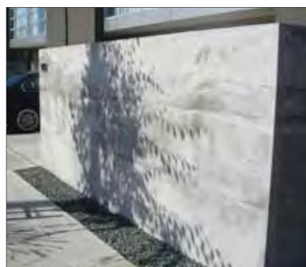
Concrete wall and french drain
