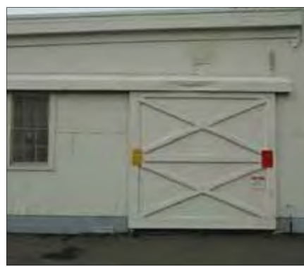
Single slider garage door with external track
