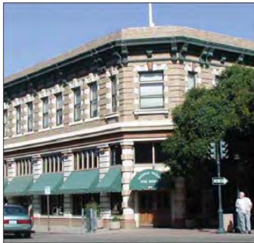
Illustrative Photo: Flex Block with shopfront frontage
