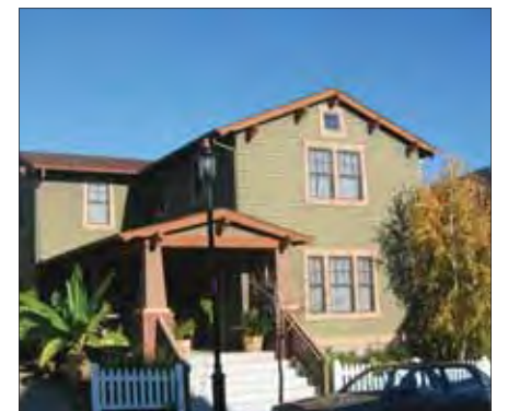
Simple gable-fronted, L-shaped form
