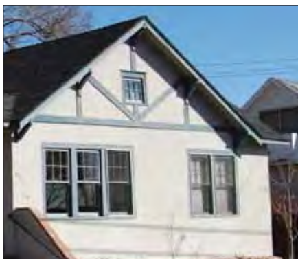
Gable ends may have decorative half-timbering
