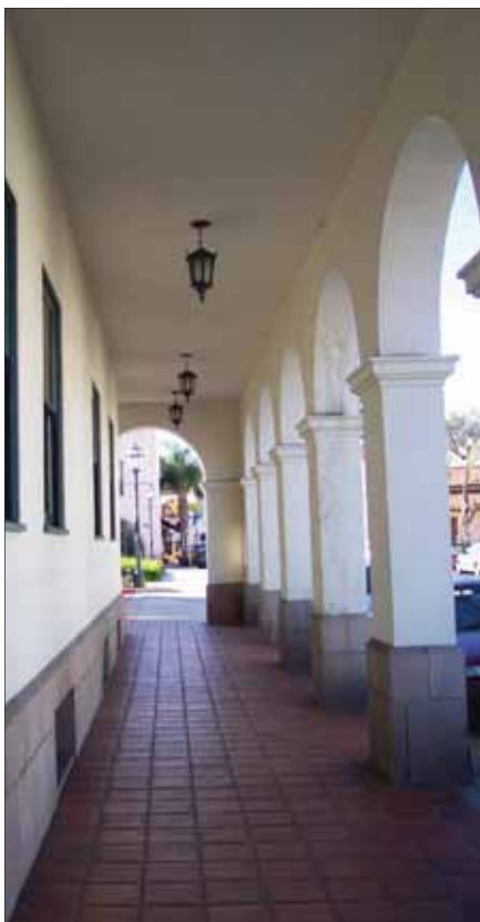
Loggia with arcade along street
