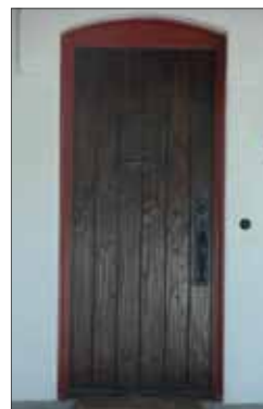
Wooden gate within arch
