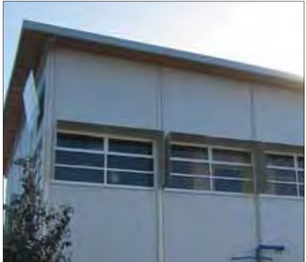
Flat roof with deep overhangs
