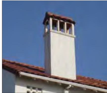
Chimney with openings and tile roof
