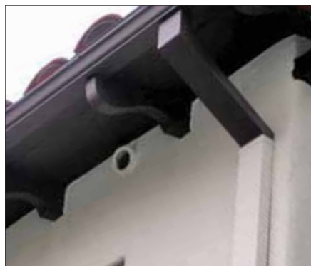
Gutter and downspout
