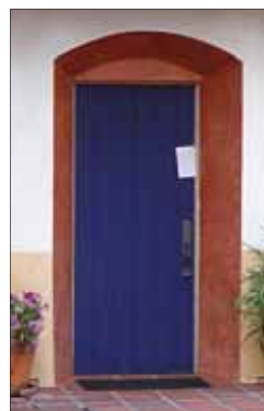
Wooden gate within arch
