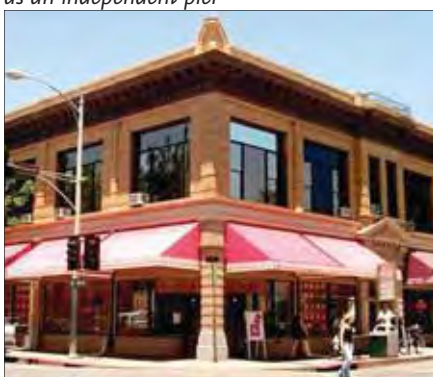
The wall below the base cornice changes material, but the base columns retain the same masonry as the primary wall
