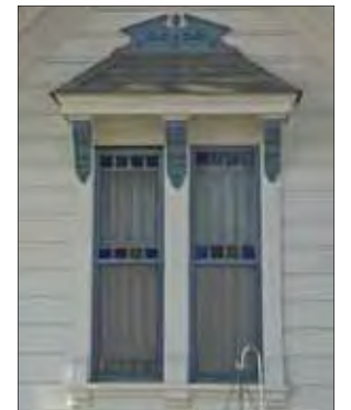
Ganged, double-hung window with decorative brackets
