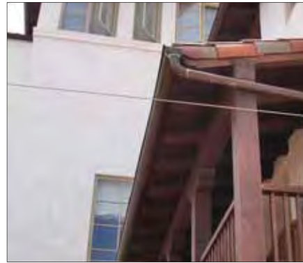
Heavy timber balcony
