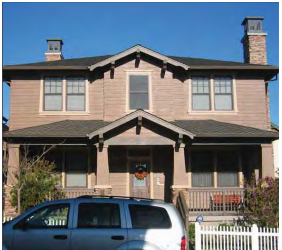
New construction with appropriate, simple massing (simple box with a few applied elements), materials, deep eaves with brackets, appropriate window sizes and porch details.
