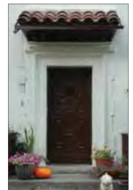
Heavy wood door with tile shed roof above
