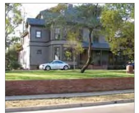
Brick retaining wall at front property line
