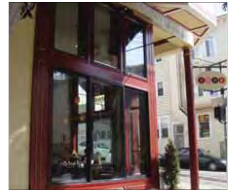
Storefront with vertical panes
