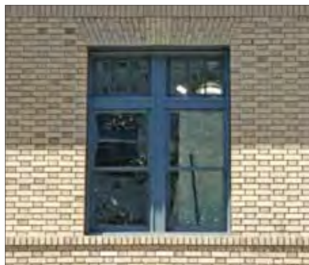
Ganged double hung windows with transom, divided by a deep mullion
