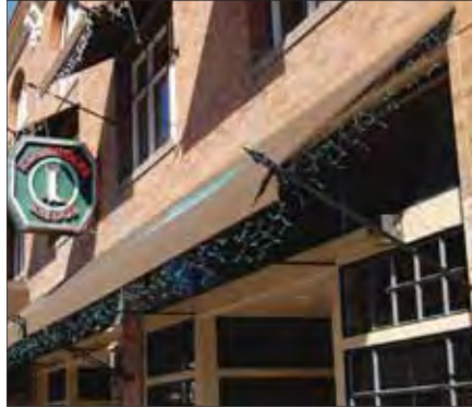
Awning that hinges above the transom windows
