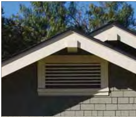
Framed vent in upper gable
