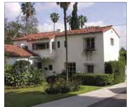
Stucco walls with windows recessed in punched openings
