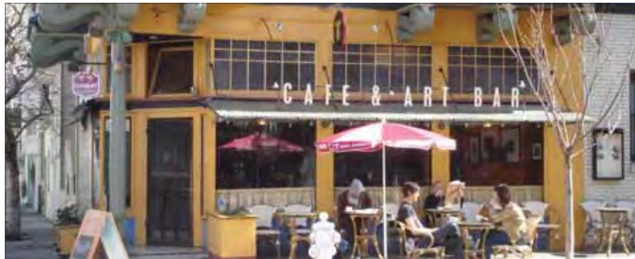
Angled corner entry storefront with transom and large, heavy brackets supporting two second-story bay windows above (bay windows not pictured)
