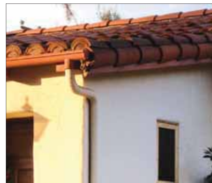
Gutter and downspout
