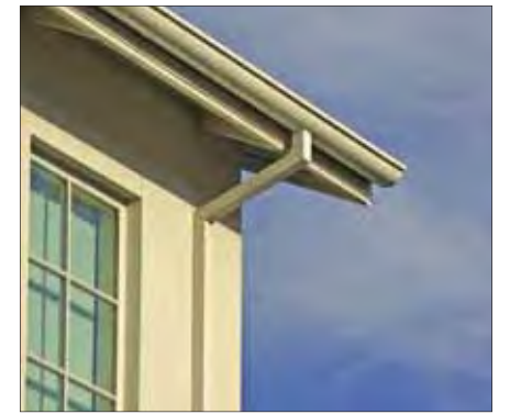
Exposed rafter tails on eave
