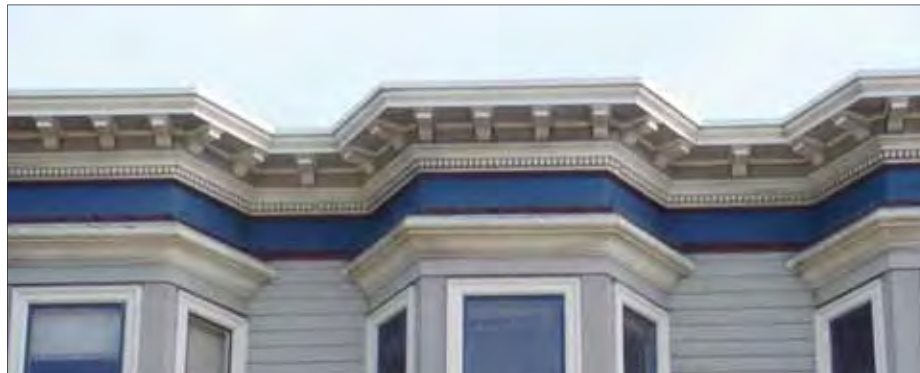
Wood siding meets the cornice, which is painted with an accent color; the cornice engages the bay windows
