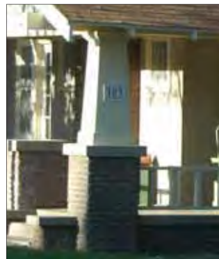
Tapered wood column with brick base
