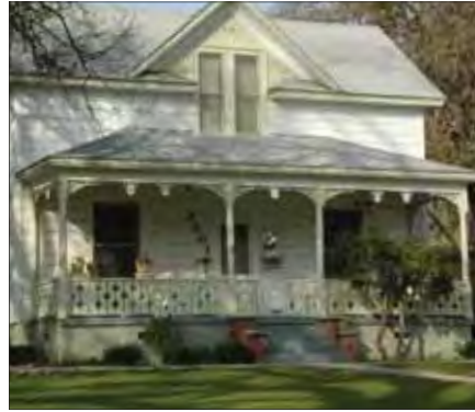
Chamfered square columns with decorative railing
