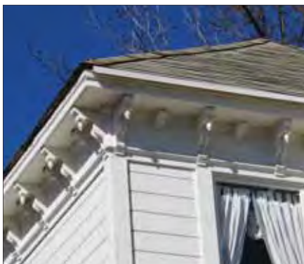
Bracketed cornice with horizontal band at the base to ground the brackets
