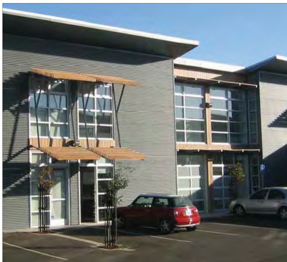
Canopy made of wooden slats on their sides providing shade but not protection from rain
