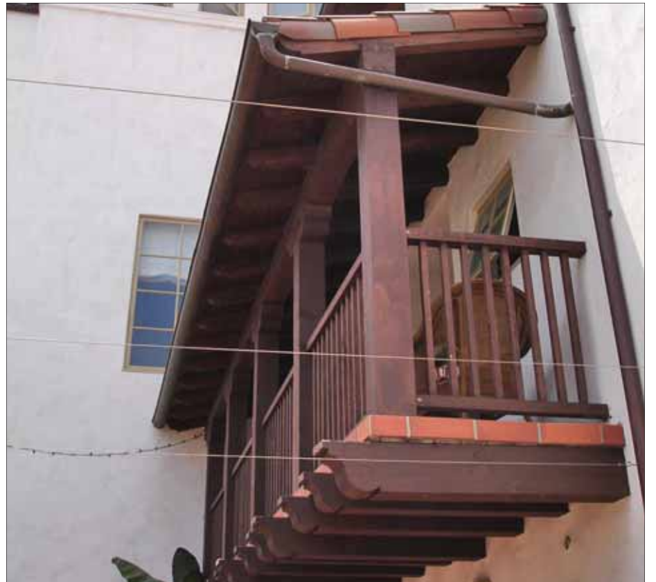
Covered wood balcony supported by heavy brackets
