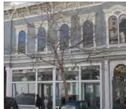
Combination of painted wood siding on the second floor and smooth stucco below
