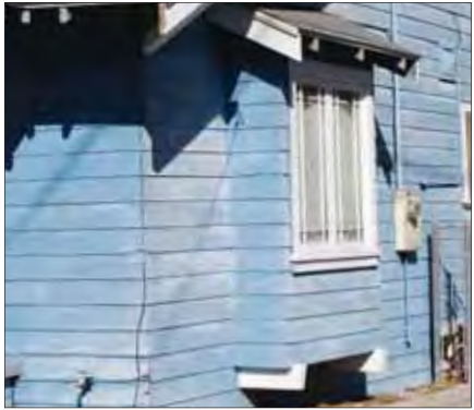
Square side bay supported by heavy brackets
