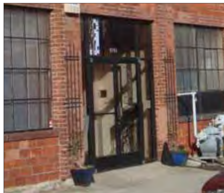
Residential entrance for warehouse lofts
