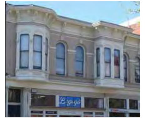
Tall, formal continuous cornice
