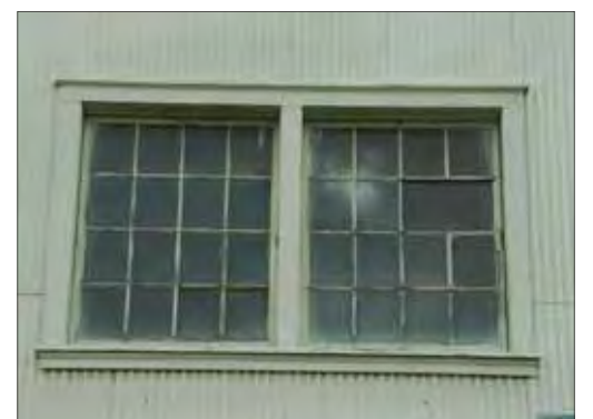
Paired fixed windows with vertical divided lites
