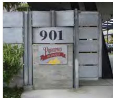
Low wall incorporates more privacy with sheet metal panels above wall
