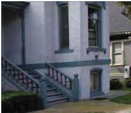
Brick veneer extends to concrete base
