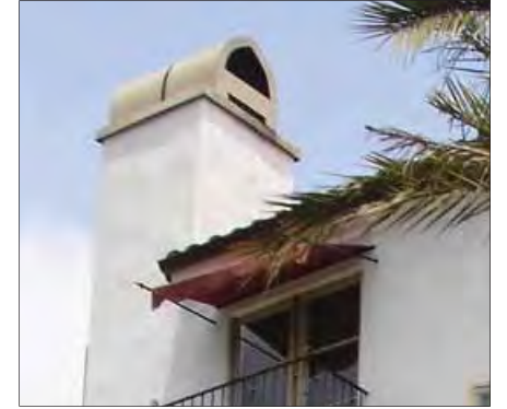
Chimney with openings and roof
