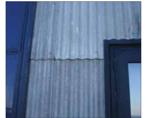
Vertical corrugated sheet metal siding
