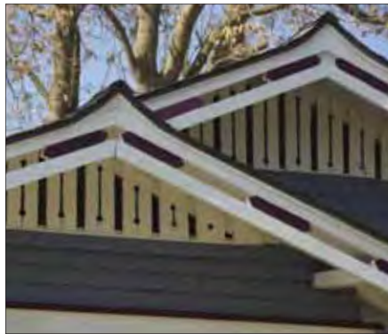
Slatted wood attic vent
