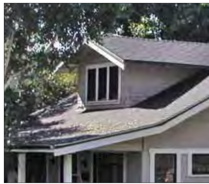
Dormer window with pitched roof
