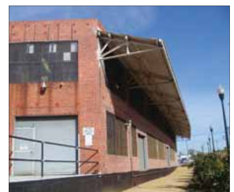
Continuous covered canopy with small steel members supporting corrugated metal roof
