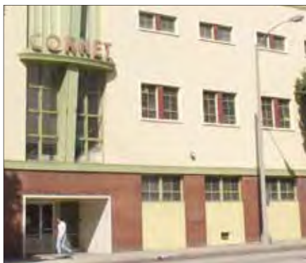
Ground floor is brick to visually act as base
