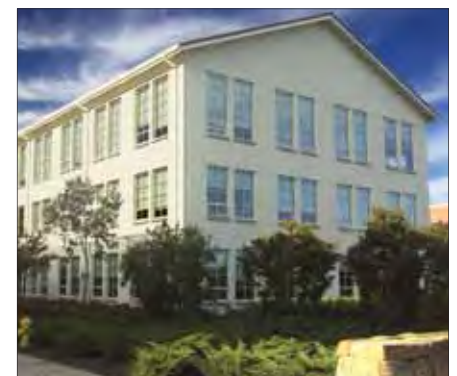
Gable end warehouse with regular openings
