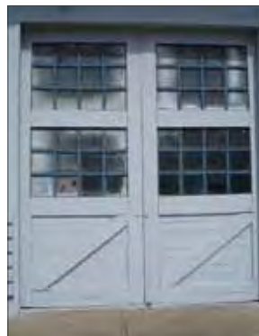
Slider doors with divided windows on internal track
