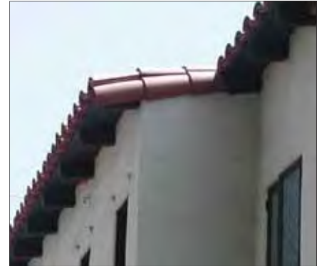
Shallow eave with large rafter tails
