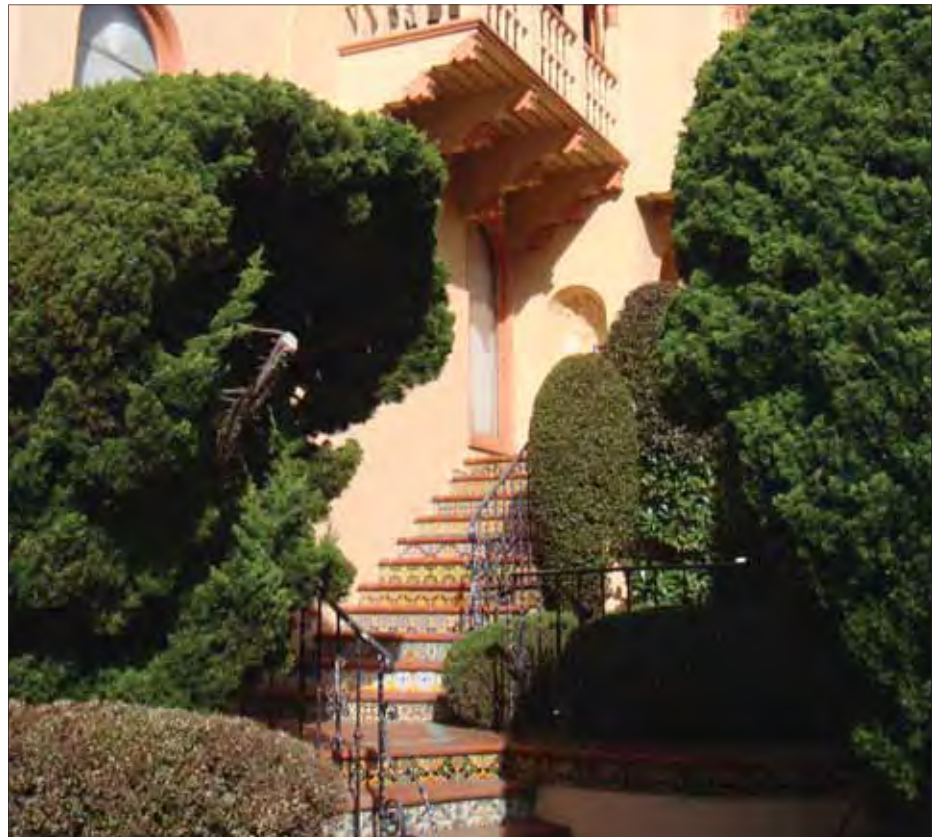
Exterior stair up to entry door; balcony above door provides some shelter.
