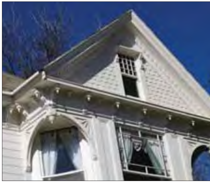
Steeply pitched gable
