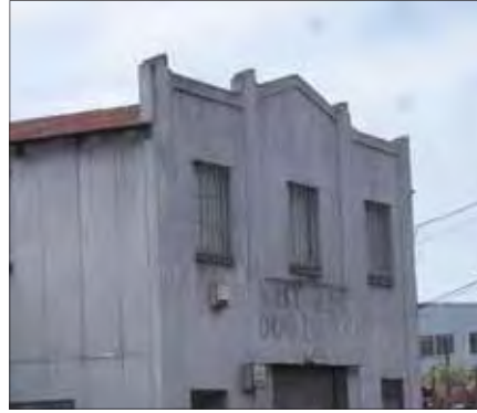
Simple warehouse with a parapet
