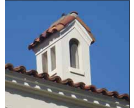
Chimney with openings and tile roof
