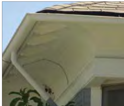
Gutter and downspout
