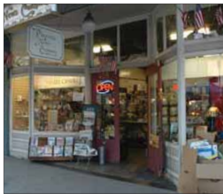
Storefront with a recessed chamfered entry and windows with transom
