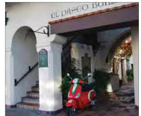
Exterior stair from street
