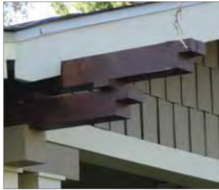
Stacked bracket supporting tall rake board
