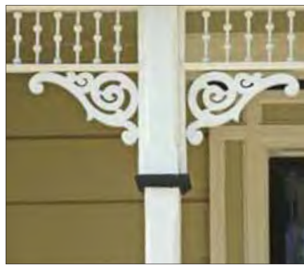
Chamfered square posts with decorative spindlework
