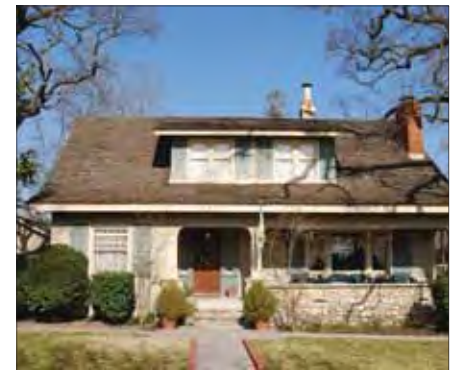
Simple cross gable form with shed dormer with an English arts and crafts character
