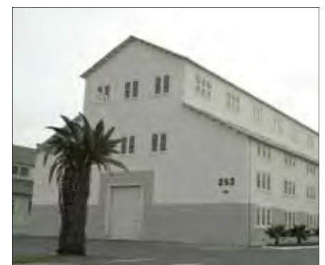
Gable end warehouse with loading door
