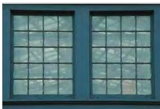
Paired fixed windows with pressed metal surrounds
