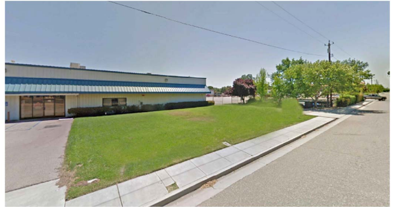
EXISTING CONDITION : SOUTH VIEW
