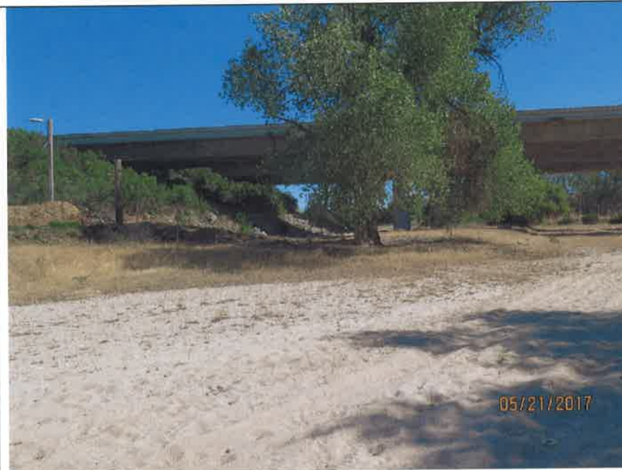
Photo 5. View south from The Ravine (light pole on the left) toward location of tramway, on the floodplain behind cottonwood trees.
