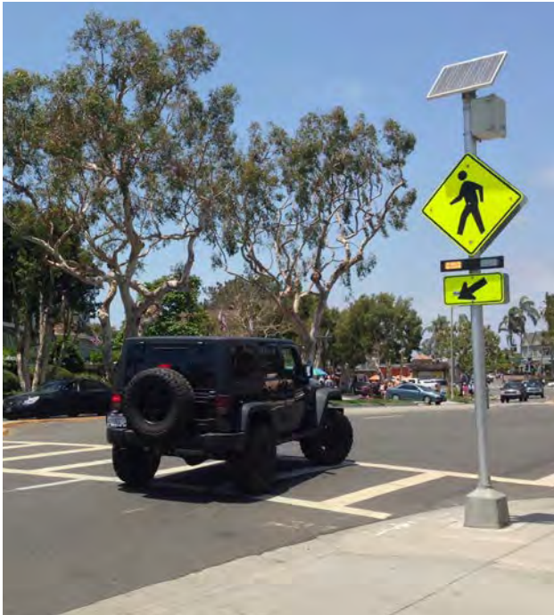
Driving Through an Activated RRFB Carlsbad, CA
