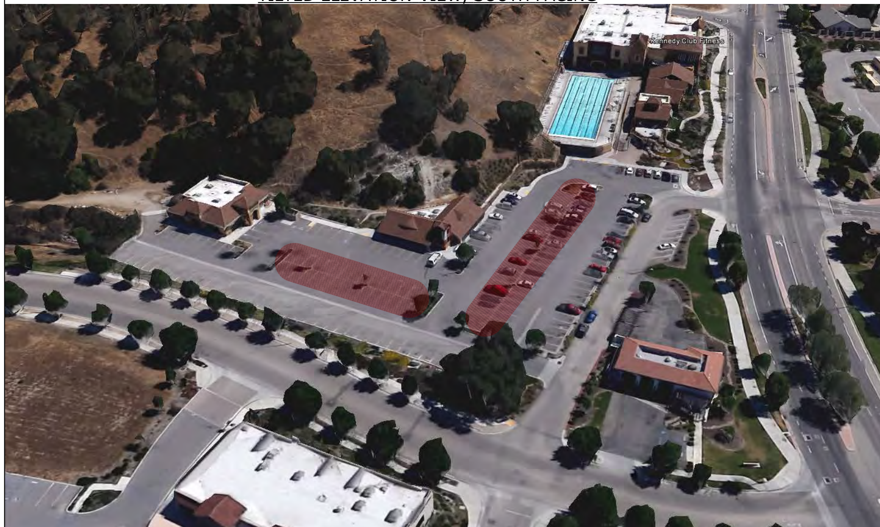
TILTED ELEVATION-VIEW, SOUTH FACING
