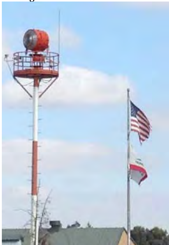
Existing 55-foot tall Beacon
