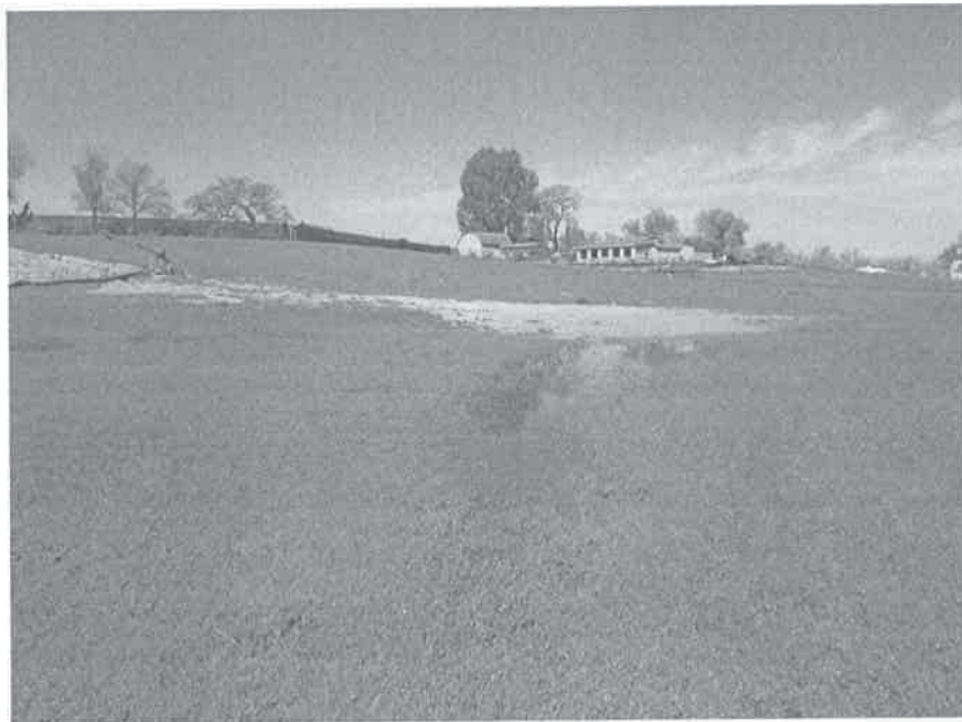
Photo 4. Ponded area east of fill soil stockpile, facing northwest. March 10, 2016.
