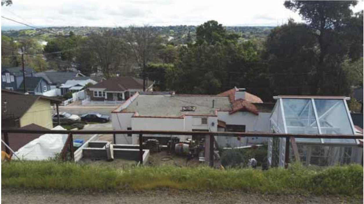
Behind 1311 Chestnut taken from fire road
