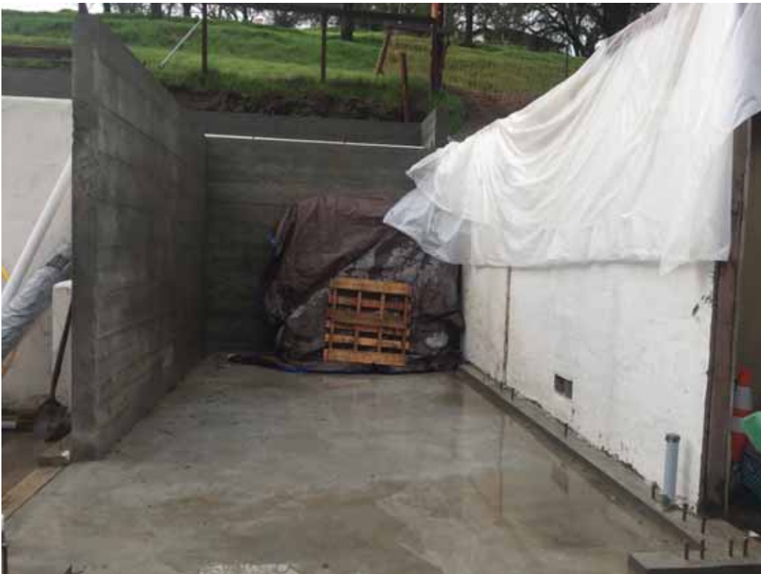
Site Photo 3: View of garage on the lower level, looking west.
