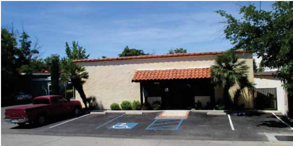
Photo 2: View of the existing building facing the rear entrance (looking north).
