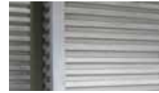
SIDING: 1 1/2" DEEP ALUMINUM WALL PANEL (MATRIX MX1.0 24 GA.) MFR: MORIN. COLOR: GALVALUME TO MATCH EXISTING
