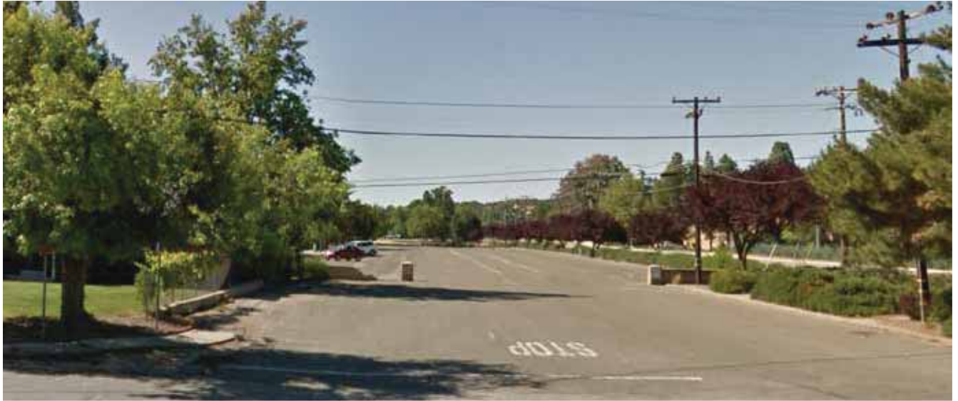
Photo #1: Looking south at the Sherwood Park parking lot from Santa Ynez Avenue.
