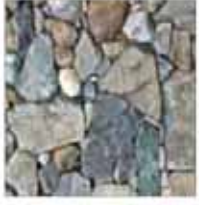
LOOSE STONE WALL
