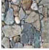
LOOSE STONE WALL
