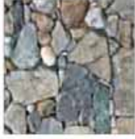
LOOSE STONE WALL
