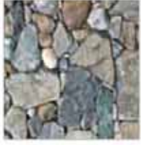
LOOSE STONE WALL
