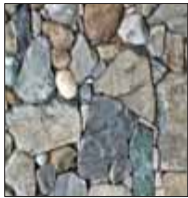
LOOSE STONE WALL
