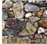
LOOSE STONE WALL
