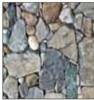
LOOSE STONE WALL
