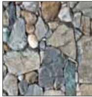
LOOSE STONE WALL
