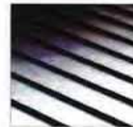
STANDING BATTAN METAL ROOF
