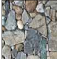
LOOSE STONE WALL
