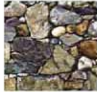
LOOSE STONE WALL
