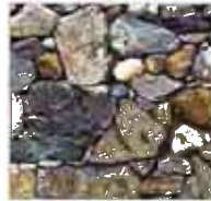
LOOSE STONE WALL
