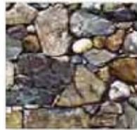
LOOSE STONE WALL
