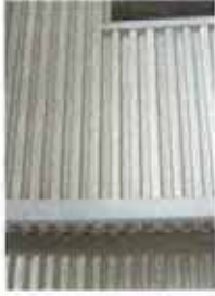
SIDING: 1 1/2" DEEP ALUMINUM WALL PANEL (MATRIX 1.0 24 GA) MFR: MORIN, COLOR: GALVALUME TO MATCH EXISTING
