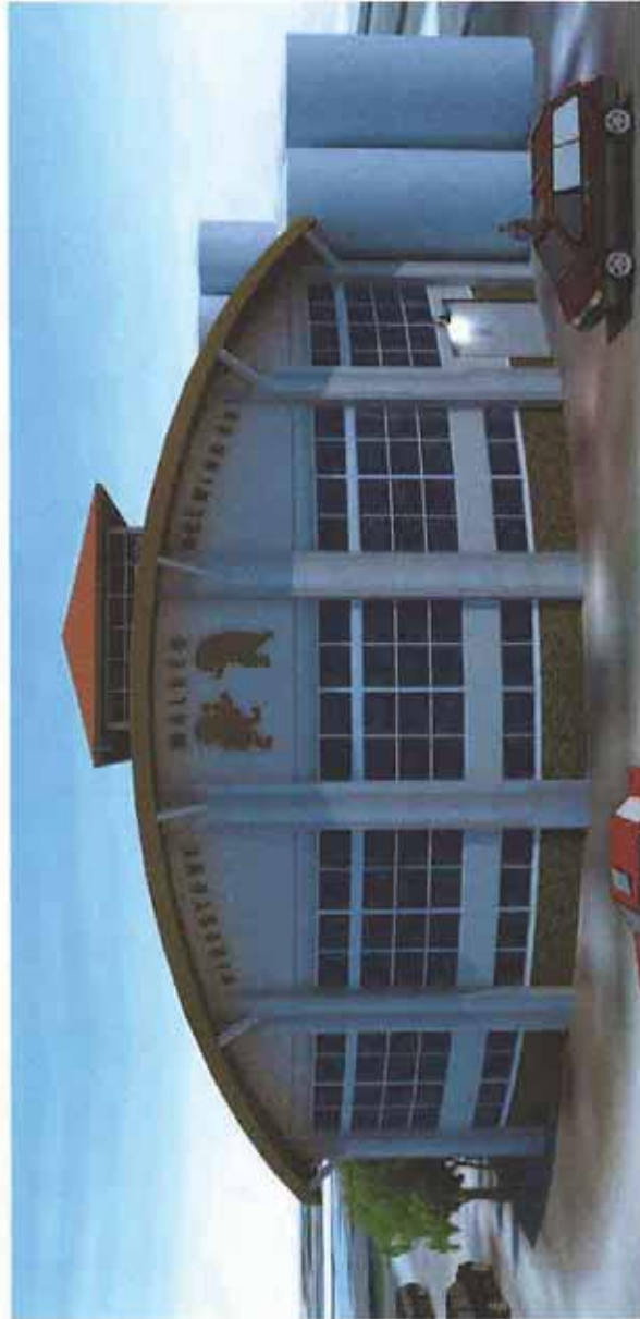
COLUMN COVERS: PRE-FINISHED SMOOTH ALUMINUM COLUMN COVERS WITH SEAM @ 36" O.C.
