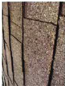
40-YEAR CLASS A FIBERGLASS ROOF.
