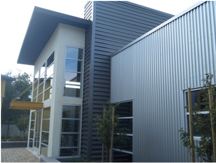
Example of Siding , BUILDING LOCATION UNKNOWN
