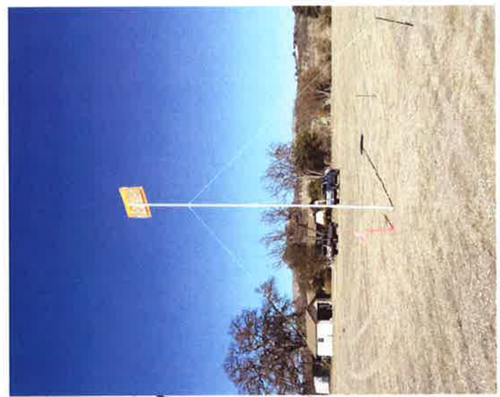
20' PYLON (ONE OF THREE PLACED AT SURVEYED BUILDING CORNERS)
