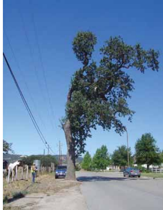
Photo 4. Tree 70 – View west on Experimental Station Road (2012 condition).
