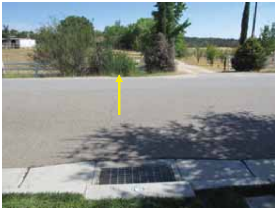
9. Stormwater inlet collects water that is carried under street toward the Property. Cattails indicated by arrow. Mulefat bush to the left, and landscape and fruit trees to the right in photo taken July 2012, view south.
