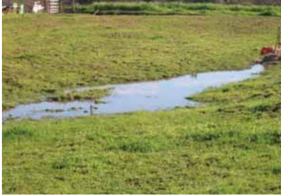
7. A small swale begins at a culvert from under Experimental Station Road on the residential parcel to the east, and continues through Tract 2696 to Highway 46 East. Standing water was present on February 28, 2005.
