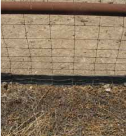
13. Typical pasture fencing with narrow openings at the lower portion of the fence. This type of fencing is difficult for many medium sized wildlife species to move through.
