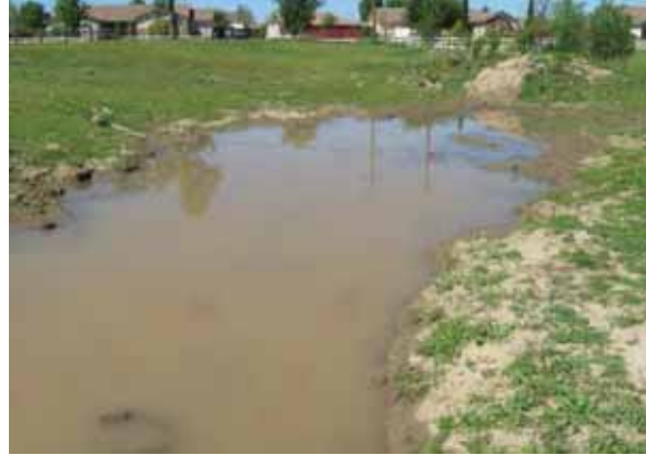
8. The swale has been altered somewhat but continues to have ponded water during the wet season. Photo taken April 20, 2012, following 1.75 inches of rain over the previous week.
