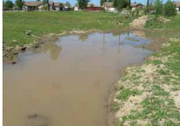
8. The swale has been altered somewhat but continues to have ponded water during the wet season. Photo taken April 20, 2012, following 1.75 inches of rain over the previous week.
