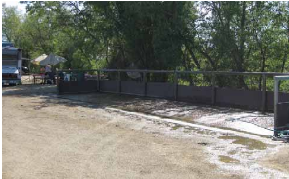
Example of wash racks in San Juan Capistrano
