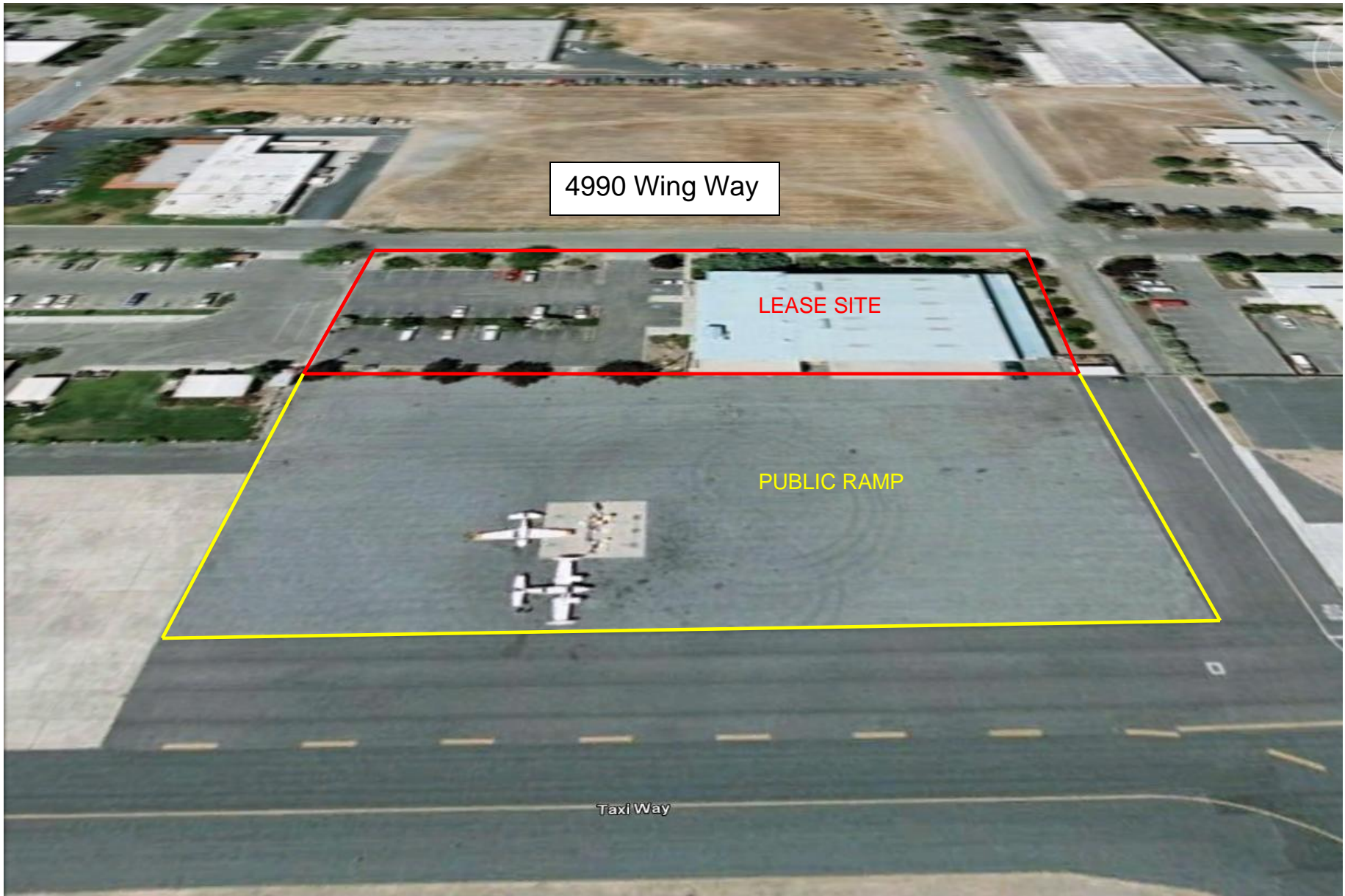
4990 Wing Way Aerial
