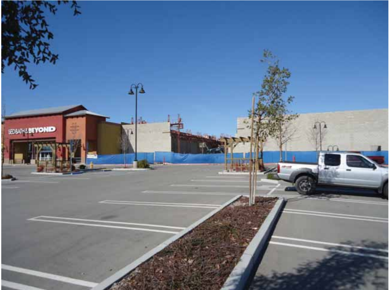
TJ Maxx, 2453 Golden Hill Road, Under Construction, Permit Issued December 20, 2011
