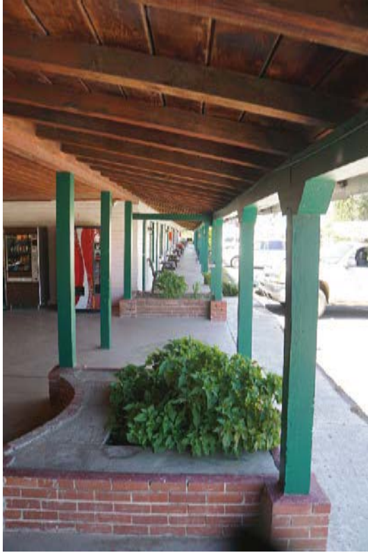
Detail of covered walkway and planter box
