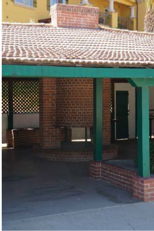
Detail of fire pit
