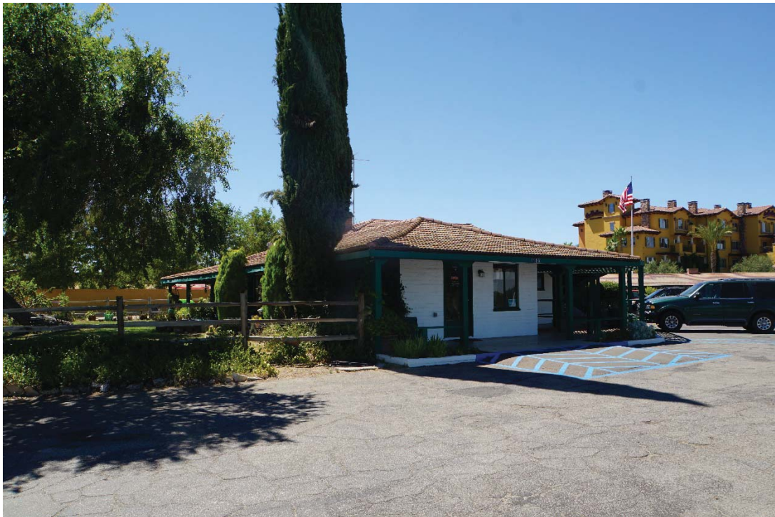
View of motel office, looking Northwest
