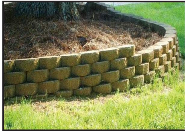
Graphic 2- Stackable Brick Wall
