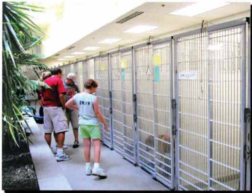
Example of new kennels in a remodeled shelter. Notice the sliding aluminum gates, the high lighting levels and sound absorbing ceiling.
