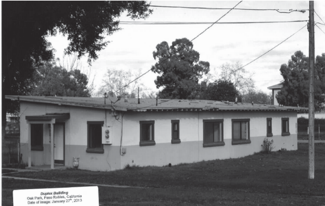
Oak Park prior to redevelopment
