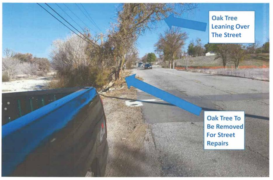
Oak tree is raising the pavement unevenly – no way to trim the roots properly since it is growing on top of the box culvert
