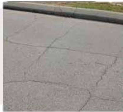
Block Cracking
