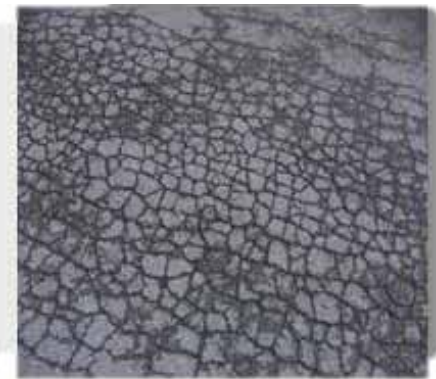
Alligator Cracking
