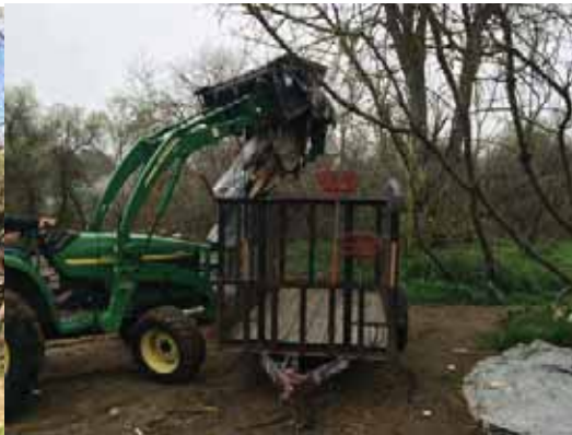
Cleanup work crew activity
