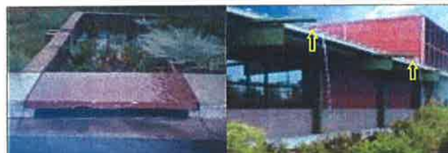
Stormdrain leading to bioretention cell
