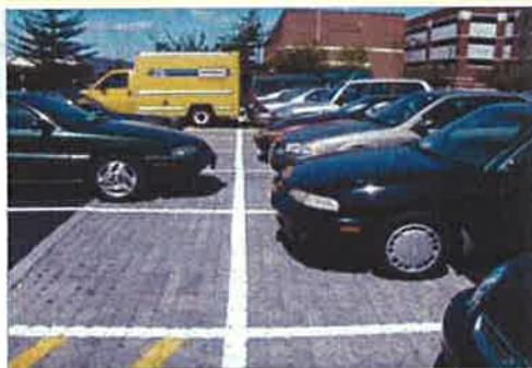
Porous pavement covers about 1/3 of each parking space in the D.C. Navy Yard parking
