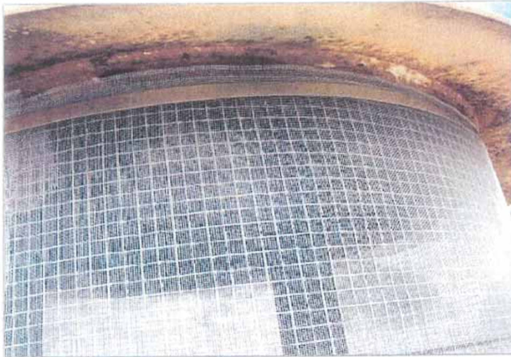
This view of the underside of the vent hood shows that the screen is in good condition and is "bug proof". Coatings are starting to fail in spots in this area with significant corrosion on the underside of the cover.
