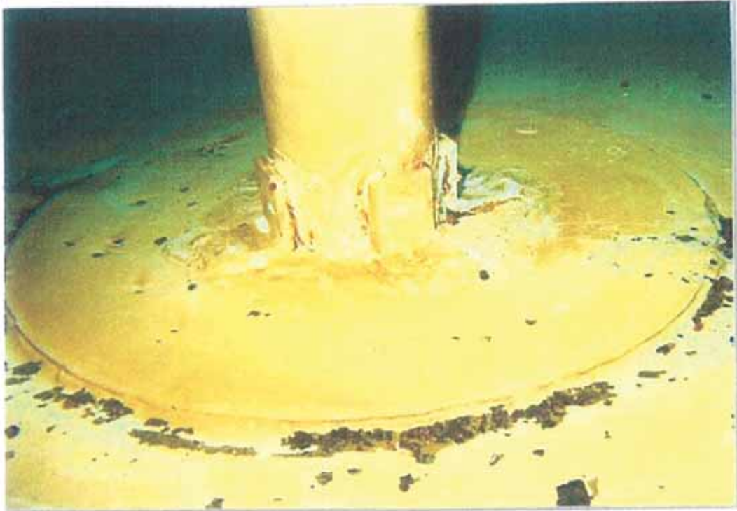
This is a view of the lower portion of the center column and base plate. Some rust points are visible on the column "clips" and sediment is visible on and around the base plate.
