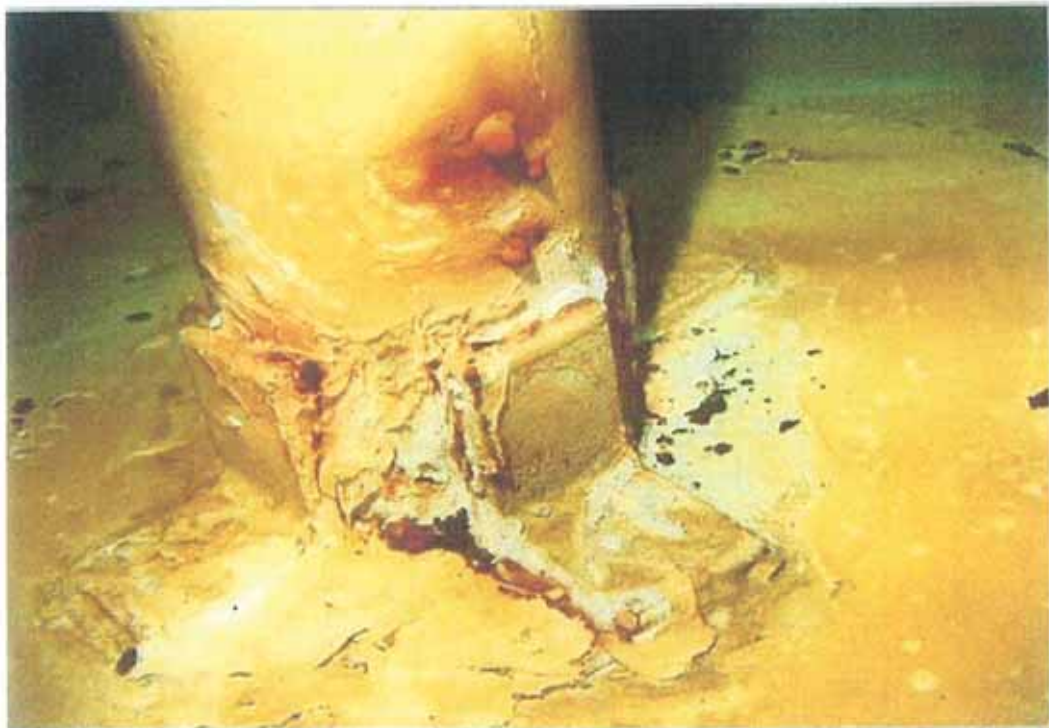
This view of the lower column shows some rust nodules that are present. The column has caulking in place to isolate inaccessible areas at the un-welded faying surfaces of the "floating" support.
