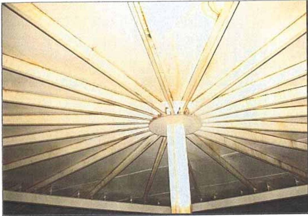
Upper center column, rafters and roof plate. Significant corrosion was present on edges of much of the structure but staining from inaccessible areas above the rafters is the source of much of the rust color.
