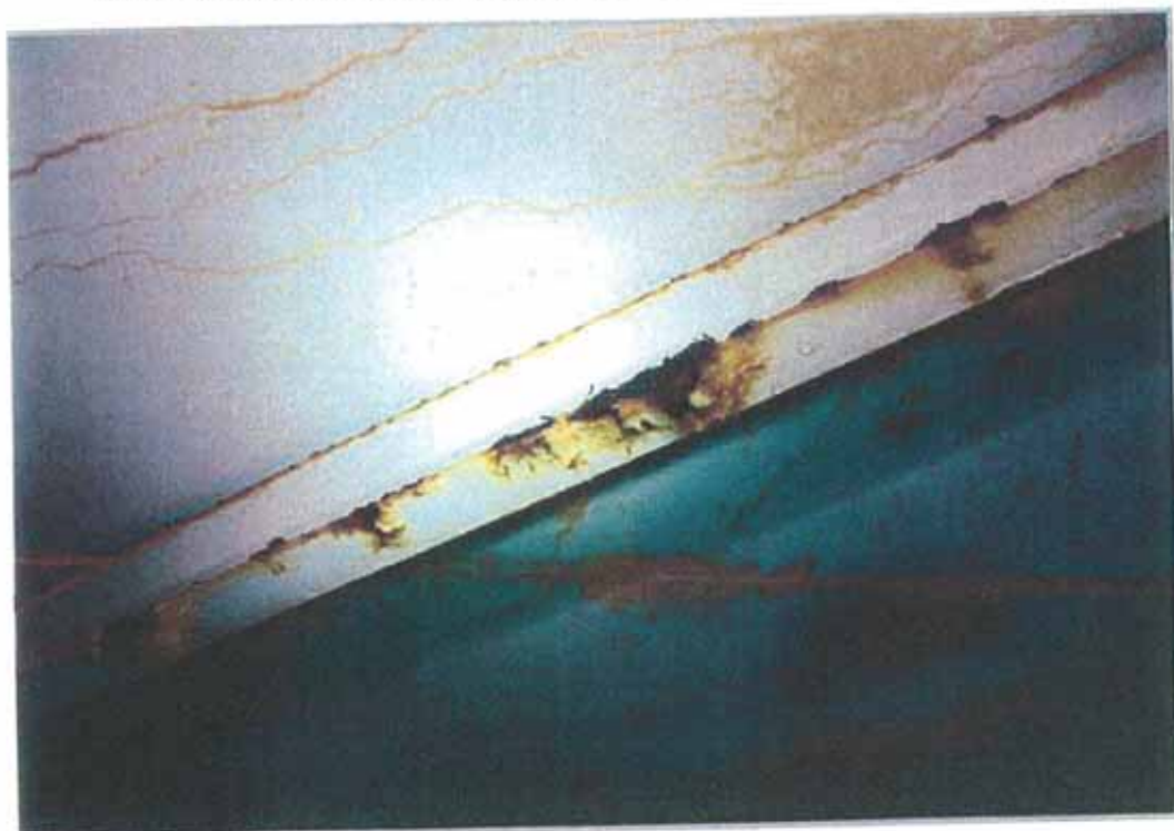
This view shows some of the aggressive corrosion that is present on the roof structure.
