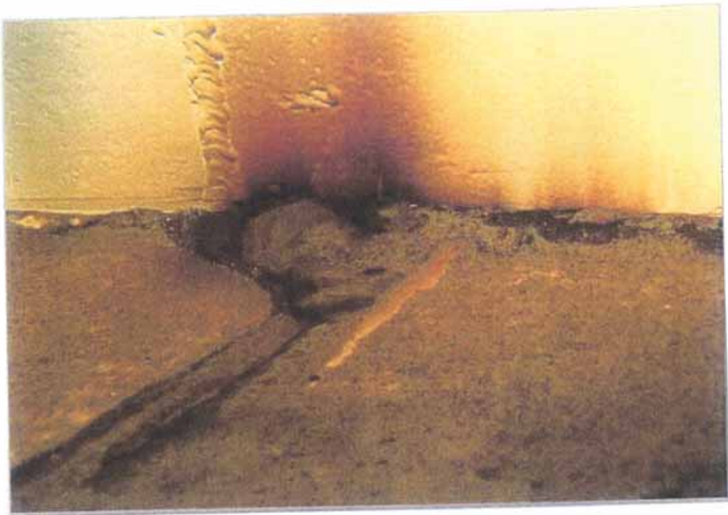
This photo of the interior bottom and shell shows the typical condition found. The coatings are cracked and corrosion is present in this area all around the tank.
