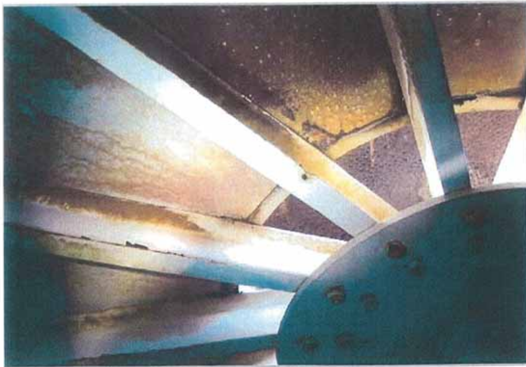
Vent area as viewed from inside the tank. Some concentrated corrosion is present on the rafters and the roof plate.
