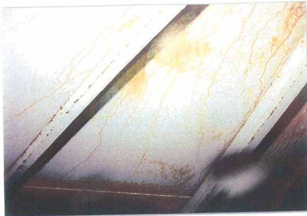
Roof plate and rafters as viewed from the water surface. This view is typical of the conditions found with general corrosion and staining on the roof plate and scattered-concentrated corrosion on the structure.
