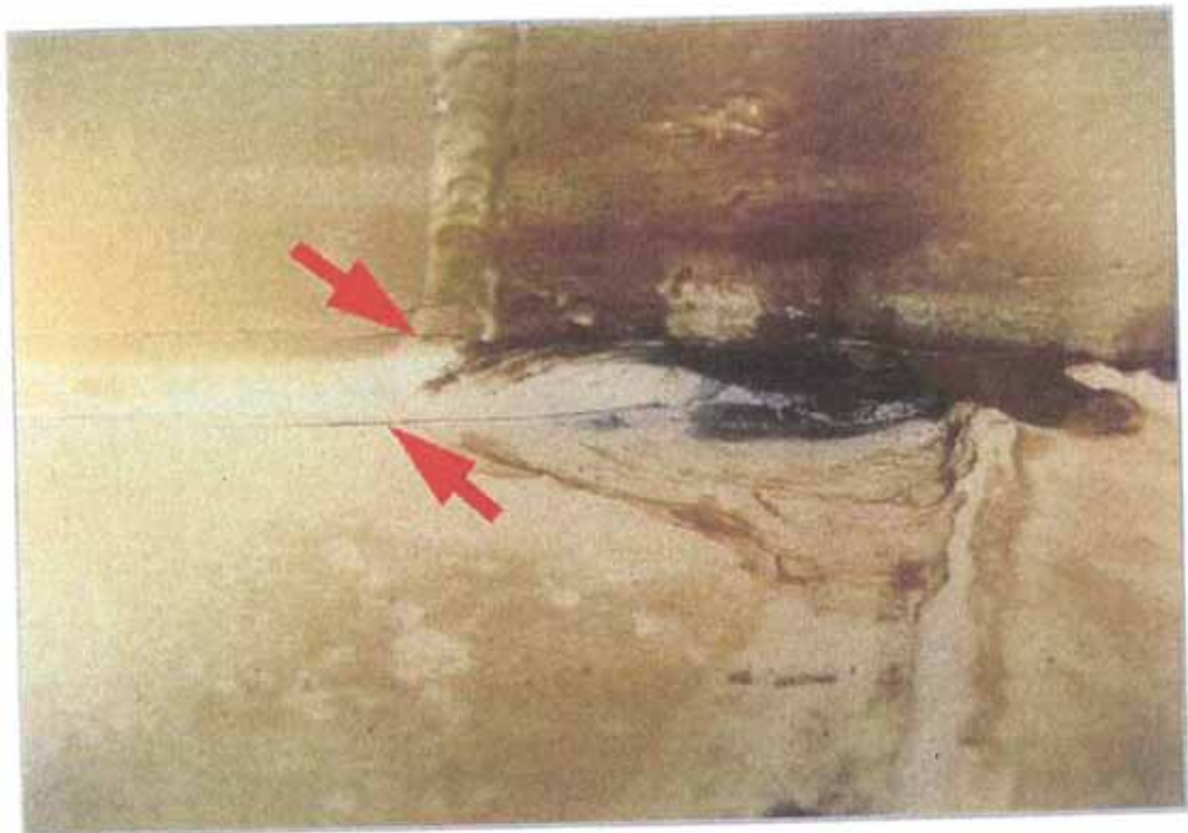
This photo shows the same area as in the top photo with the sediment removed. The rust is propagating from the cracks in the coating (arrows).
