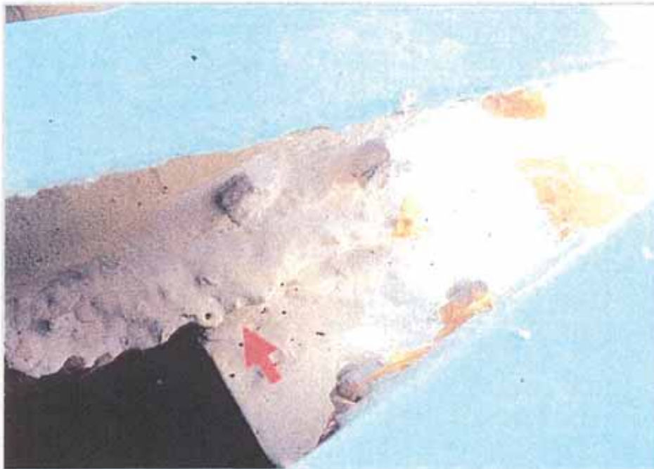
Severe metal loss due to corrosion at area of high shear load has significantly reduced the strength of the roof structure.
