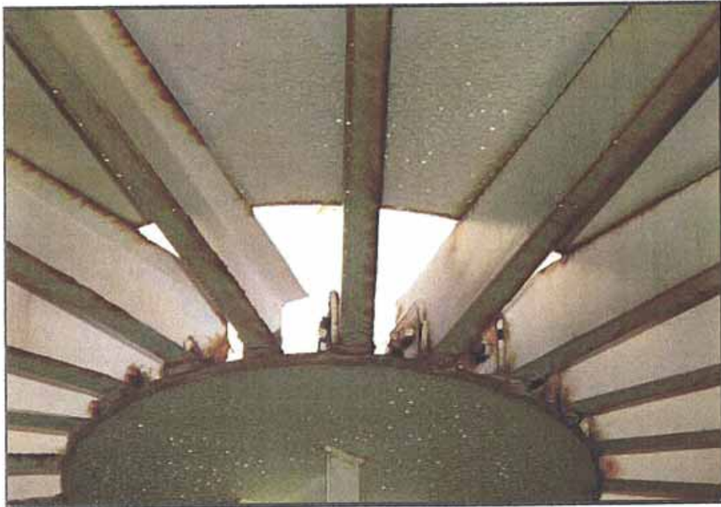
Close view of the area shown in the top photo. Significant corrosion is present around the bolts and attachment clips.
