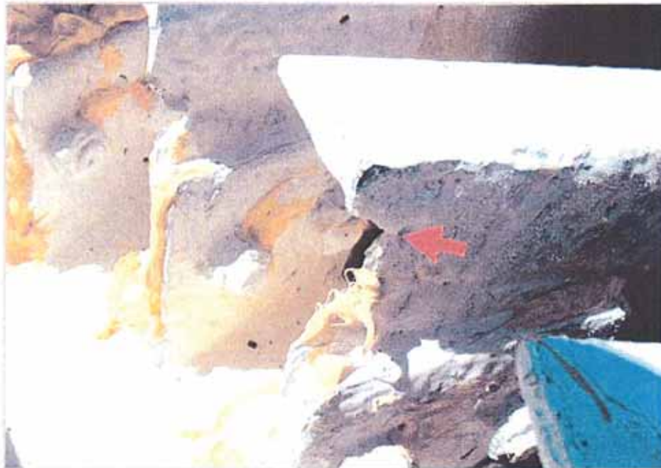
Severe metal loss due to corrosion at rafter ends has significantly reduced edge distance of structural bolting.
