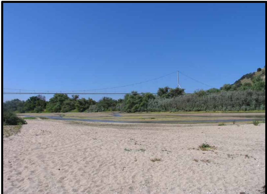
Photo Point 2 Description: Pipeline Direction: SW GPS: N 35.36339 W 120.41325
