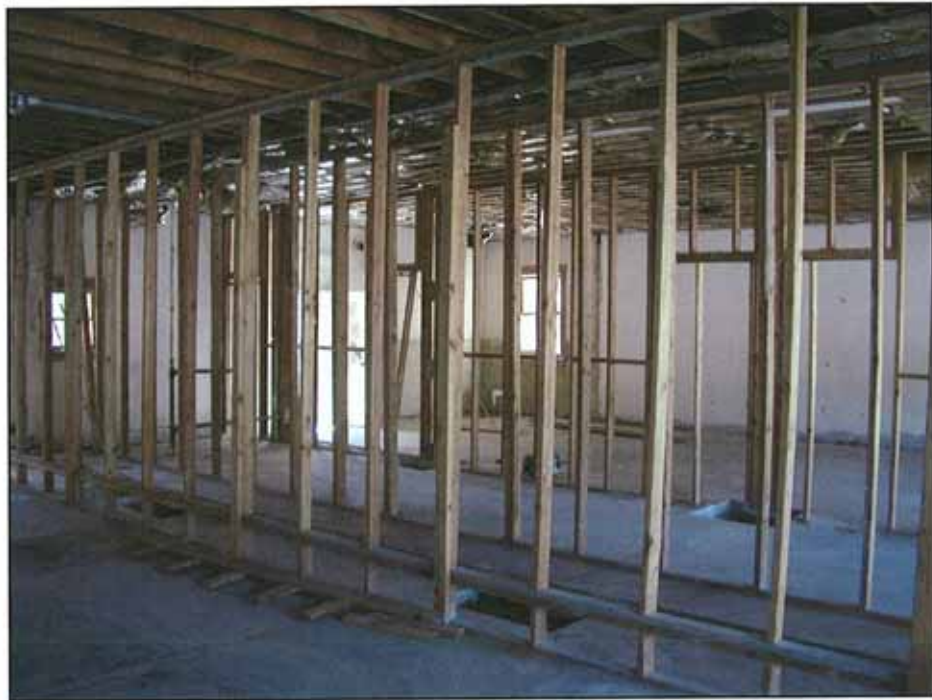
Figure 9: Interior of Commercial Building Looking SE (July 2009)
