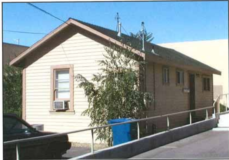
Figure 16: East & North Facade (July 2009)
