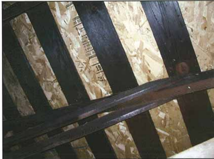
Figure 18: Rafters And OSB Plywood Roofing (July 2009)
