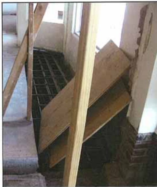
Figure 10: Commercial Building Uncompleted retrofit (July 2009)
