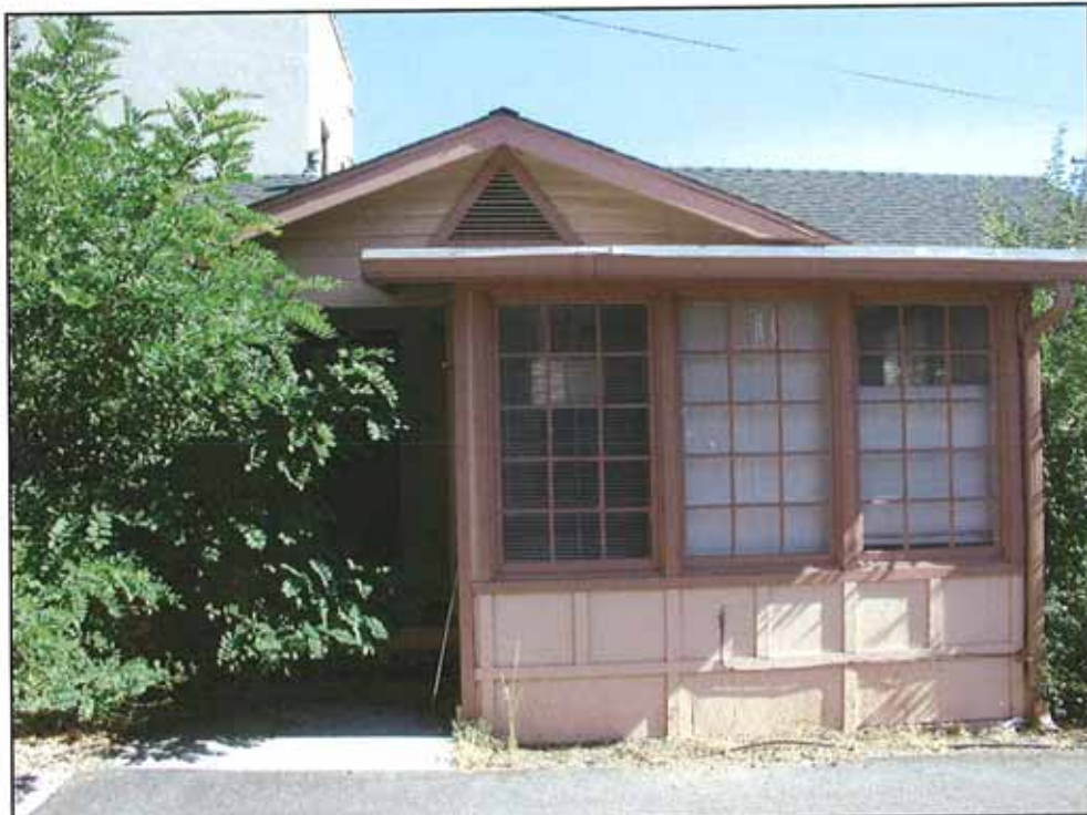
Figure 14: 1522 Spring Street South Facade (July 2009)
