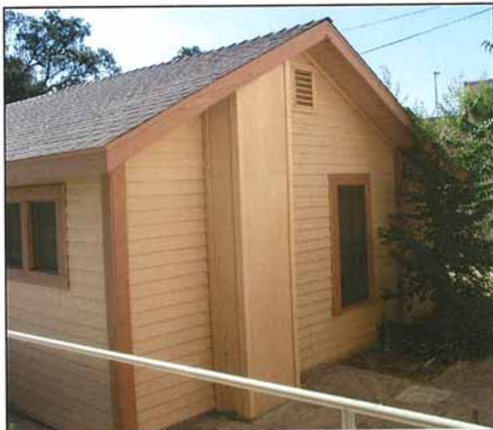
Figure 17: West Facade (July 2009)
