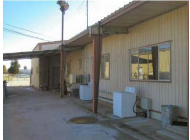
Exterior view of building rear
